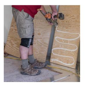
**Groove Alignment Tip.** Cut small pieces of the 1/2" PEX pipe to use as groove alignment for the boards. Step or pound these tubing guides into the boards to align them.
